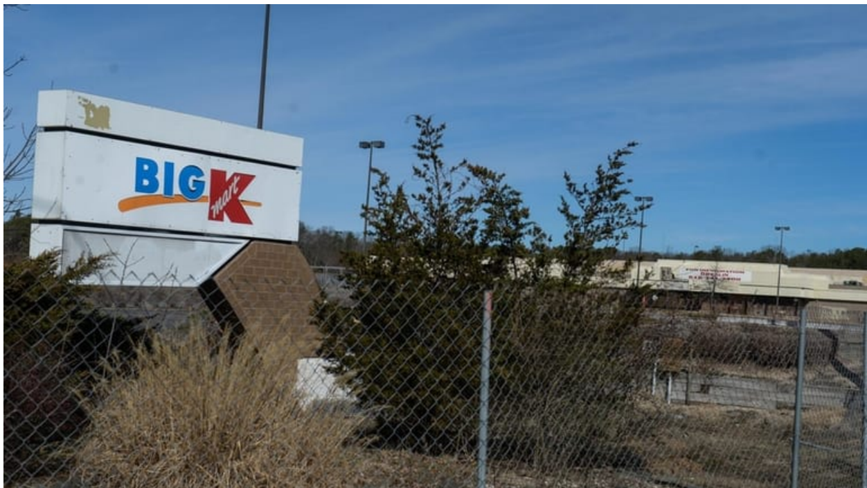
The closed store as it appeared in March 2016, just before it was demolished. Credit: Steve Pfof
